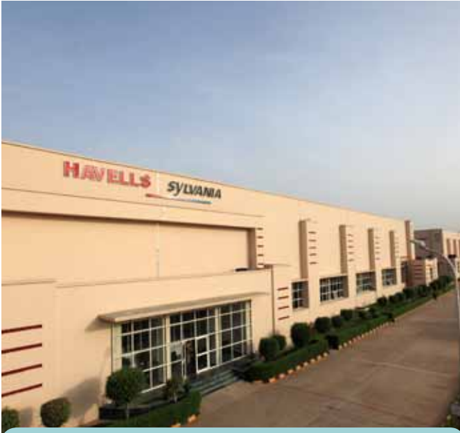
Neemrana Lighting Plant
